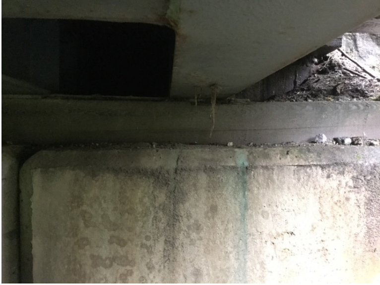
Upstream right bank sill condition
