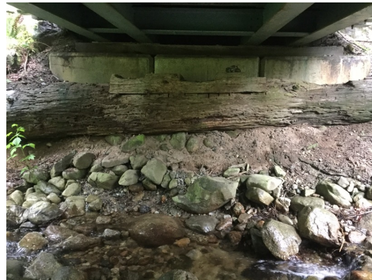
Right Bank Abutment when facing downstream
