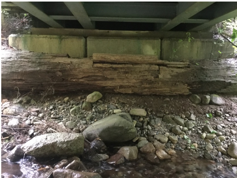
Left Bank Abutment when facing downstream
